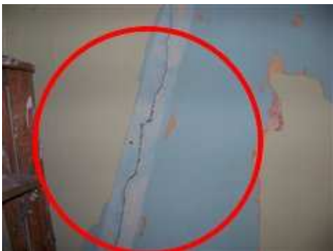
Photo 42 the plaster in th front upstairs bedroom has cracks and will need to be replaced.It appears to be superficial and not structural
